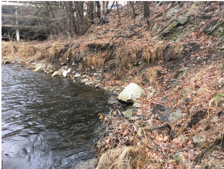
Photo 5. Former location of southern segment of Wetland 3 that has been since replaced by the revised Norwalk River channel, view to the north. Stantec. March 25, 2021.
