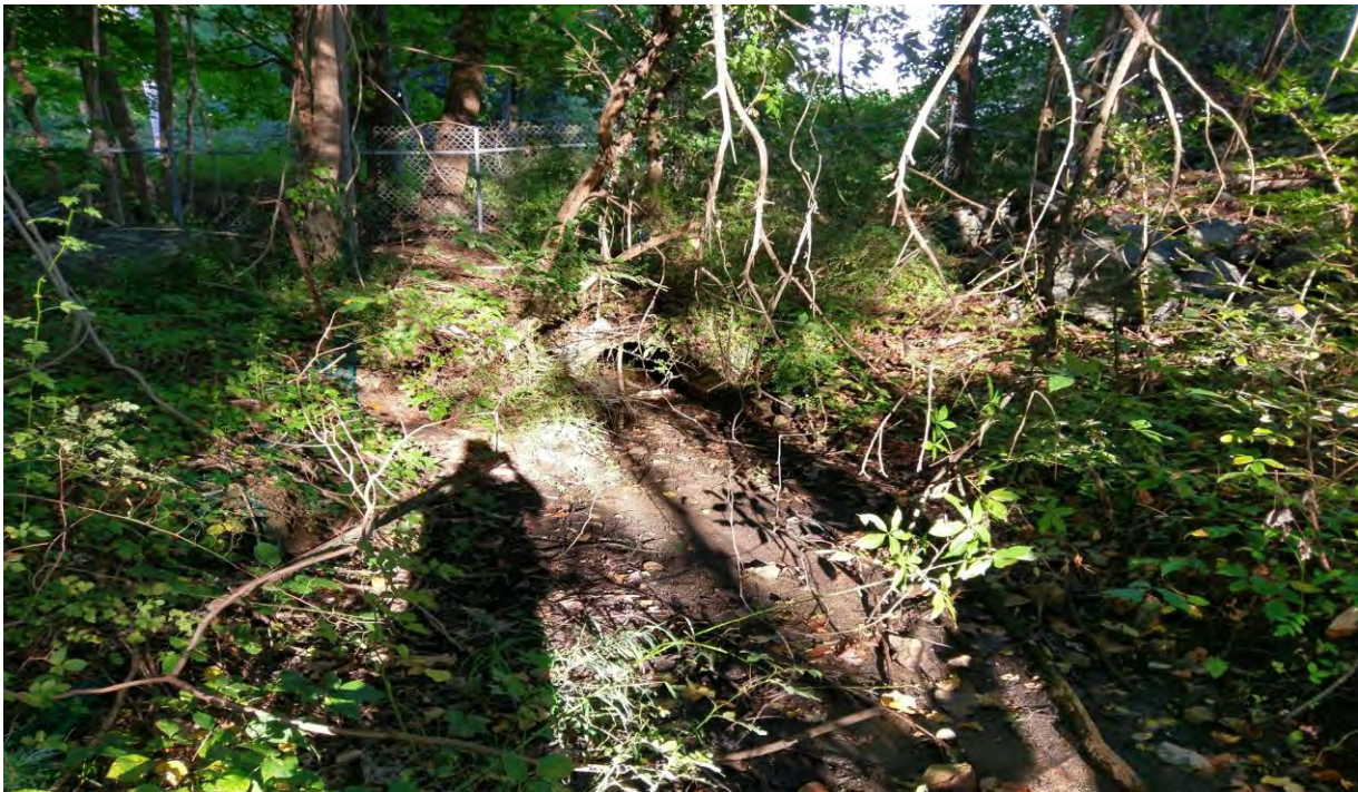
PHOTO 30: View of INT 8, looking east towards Perry Avenue, note culvert is partially buried.
