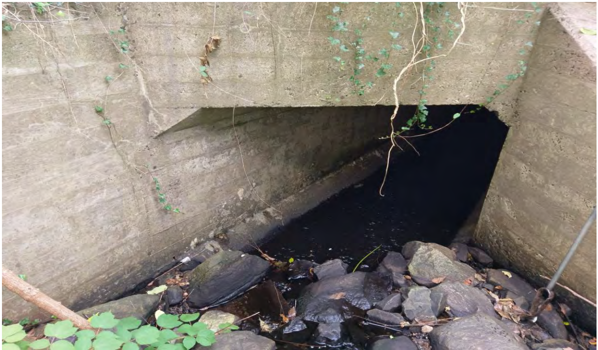
PHOTO 3: View of PER 1 box culver inlet north of Route 15 southbound.
