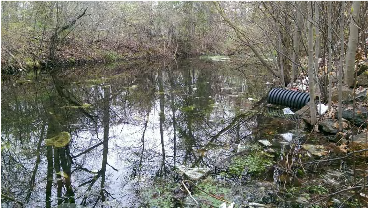
PHOTO 39: View of stormwater basin located east of Wetland 1. Note lack of vegetation in the basin, large amount of plastic in the water, and plastic corrugated pipe.
