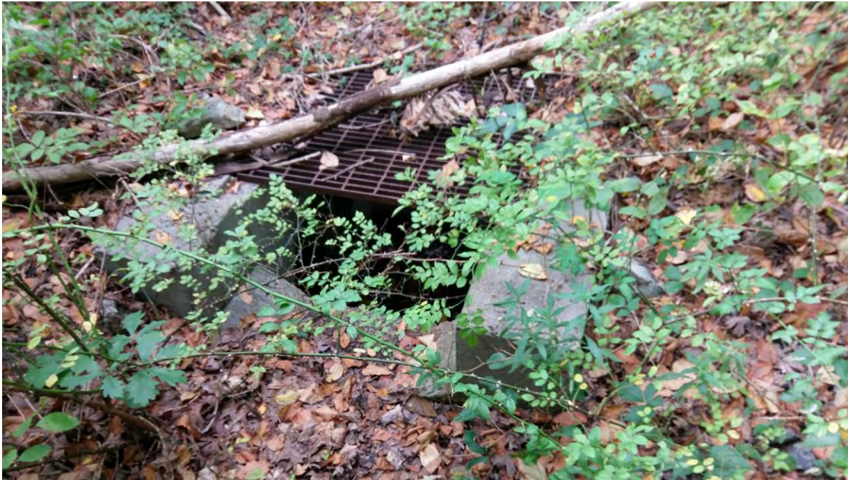
PHOTO 29: View of catch basin downstream of INT 7.
