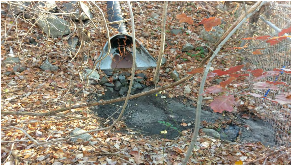
PHOTO 33: View of INT 10 pipe outfall, looking south towards Route 15 embankment.
